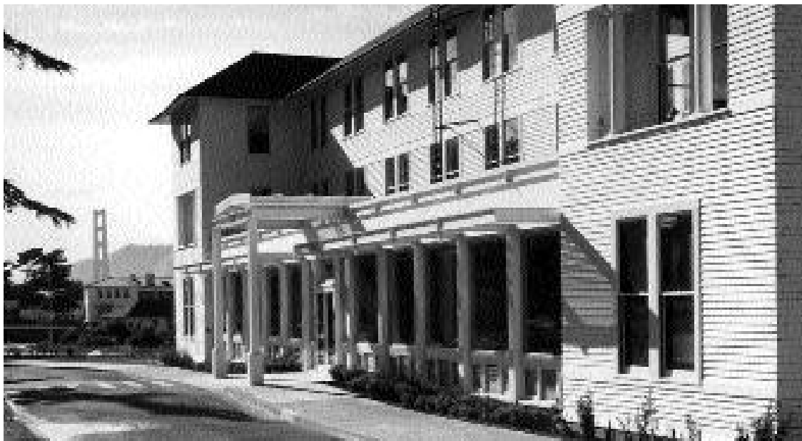
The Tides Foundation's Thoreau Center for Sustainability in San Francisco's Presidio National Park currently houses more than 50 organizations working in the areas of social, environmental and economic sustainability and is itself entirely self-sufficient because of the rents it receives
